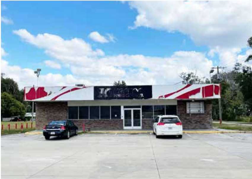
Existing Structure on South Summit Street and Prospect Street
