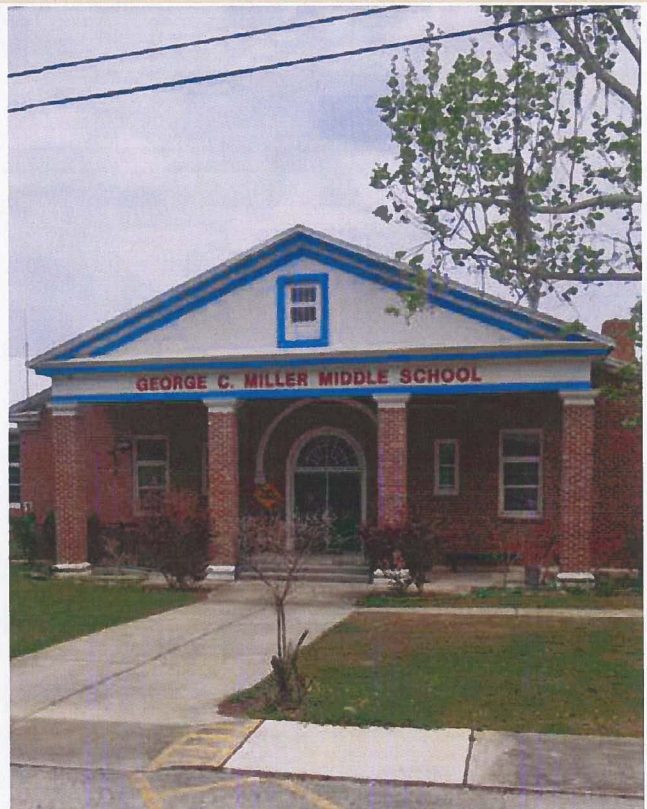
Former Middle School Site on South Prospect Street in Crescent City
