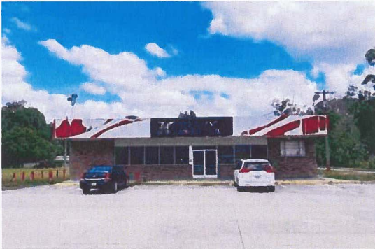
Existing Structure on South Summit Street and Prospect Street
