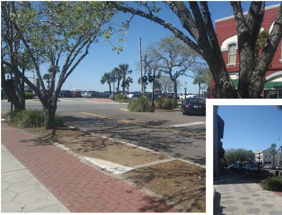
Existing concrete sidewalk can be reused and combine with various paver systems that will allow rain water to percolate back into the ground and away from street and walkways.
